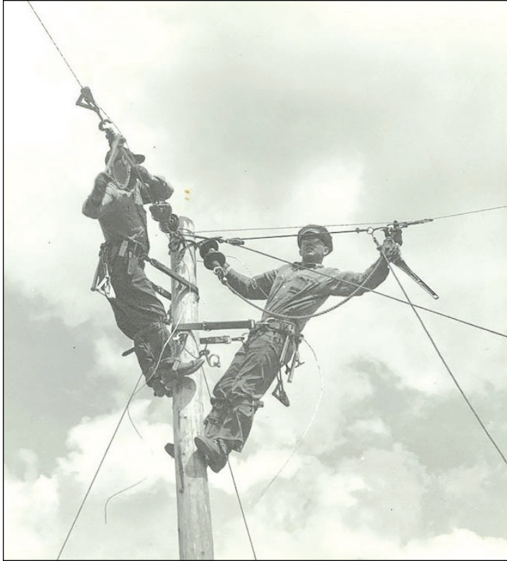
Early linemen work on Pierce Pepin electric lines.
