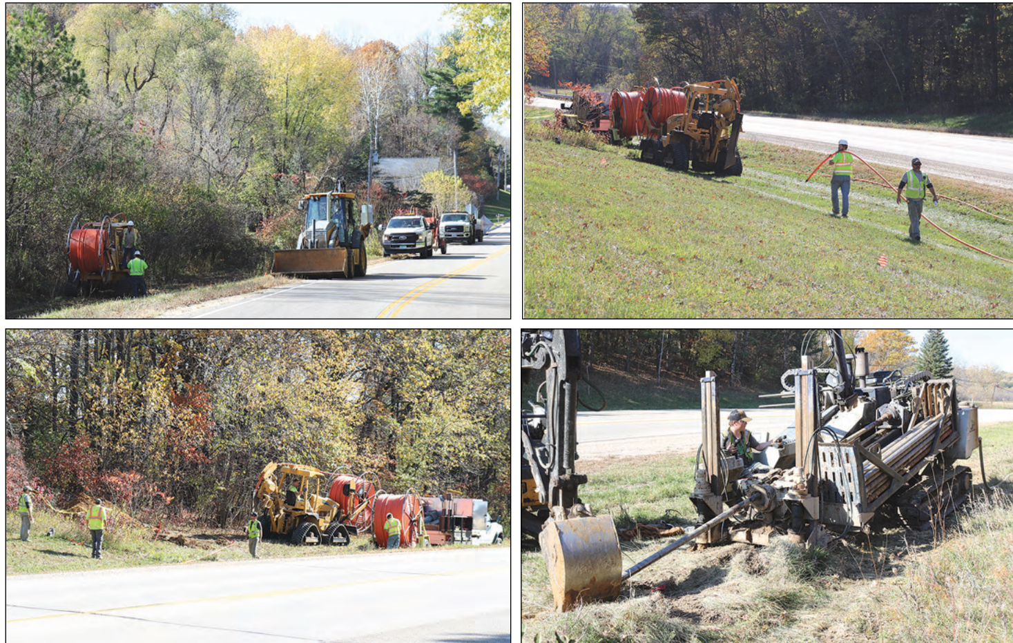
Contractors arrived in mid-September and began construction of the underground fiber lines. Fiber optic cable will be pulled through the piping they have installed. Photo courtesy of Pierce Pepin Cooperative Services/SwiftCurrent Connect
