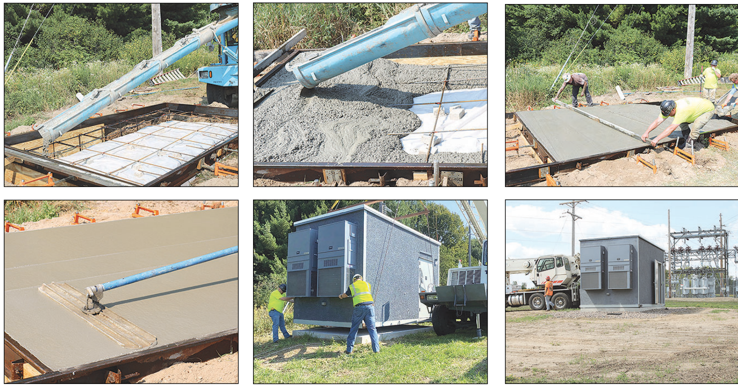
Communication huts were installed at the Beldenville and El Paso substations. Foundations were poured at each site for the huts which were lifted onto the pads using cranes. Photo courtesy of Pierce Pepin Cooperative Services/SwiftCurrent Connect
