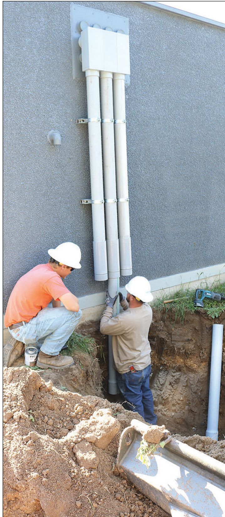
Ryan Meyer (right), PPCS master electrician, is responsible for connecting the communication huts at the Beldenville and El Paso substations with the help of seasonal worker Tyler Bee. Photo courtesy of Pierce Pepin Cooperative Services/SwiftCurrent Connect
